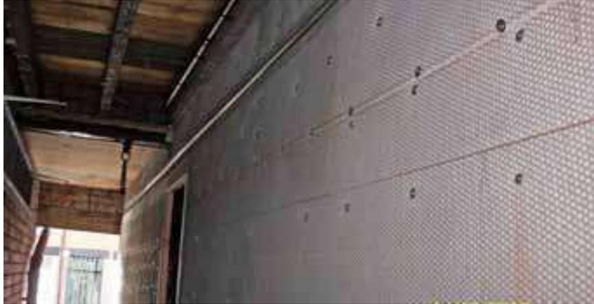
**Image of externally insulated enclosed passage**
