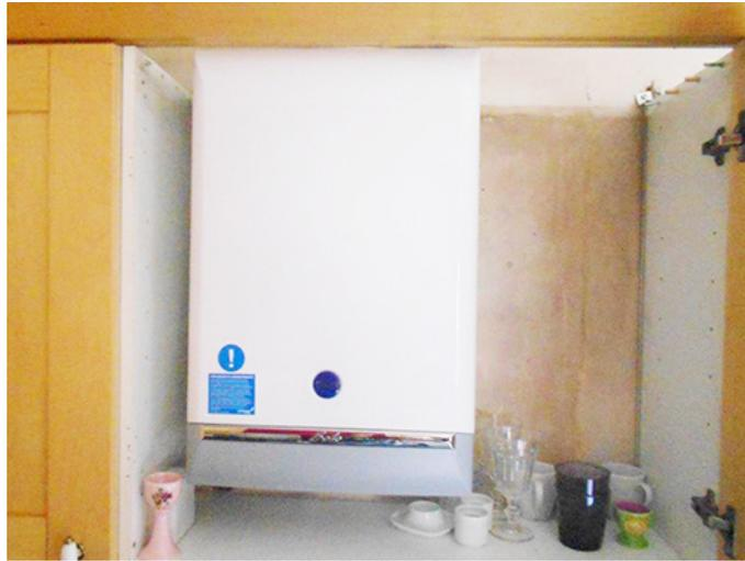
**The Akhtar’s new boiler, an A Rated Baxi Solo 15 HE A, is very compact - it is small enough to fit inside one of the family’s kitchen cabinets.**
