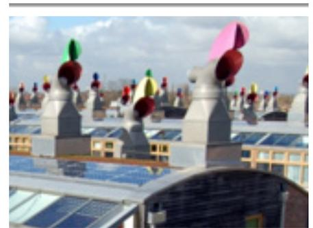
Wind-driven ventilation with heat recovery
