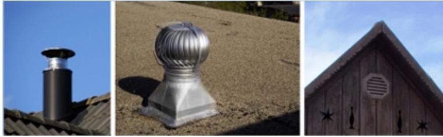
Roof vents: open stack, turbine, and gable vents
