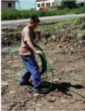
Horizontal collector pipes can be laid in various orientations. These are examples in domestic installations.
