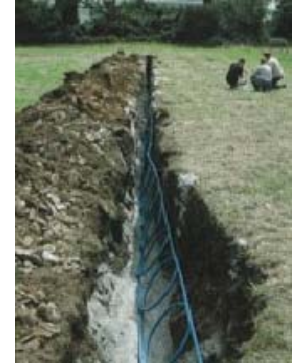
Horizontal collector pipes can be laid in various orientations. These are examples in domestic installations.
